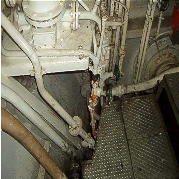
Pipes corroded
